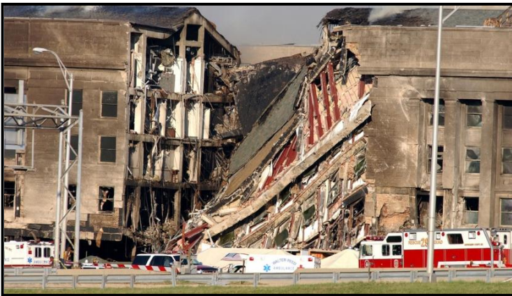
Damage to the Pentagon on 9/11.
